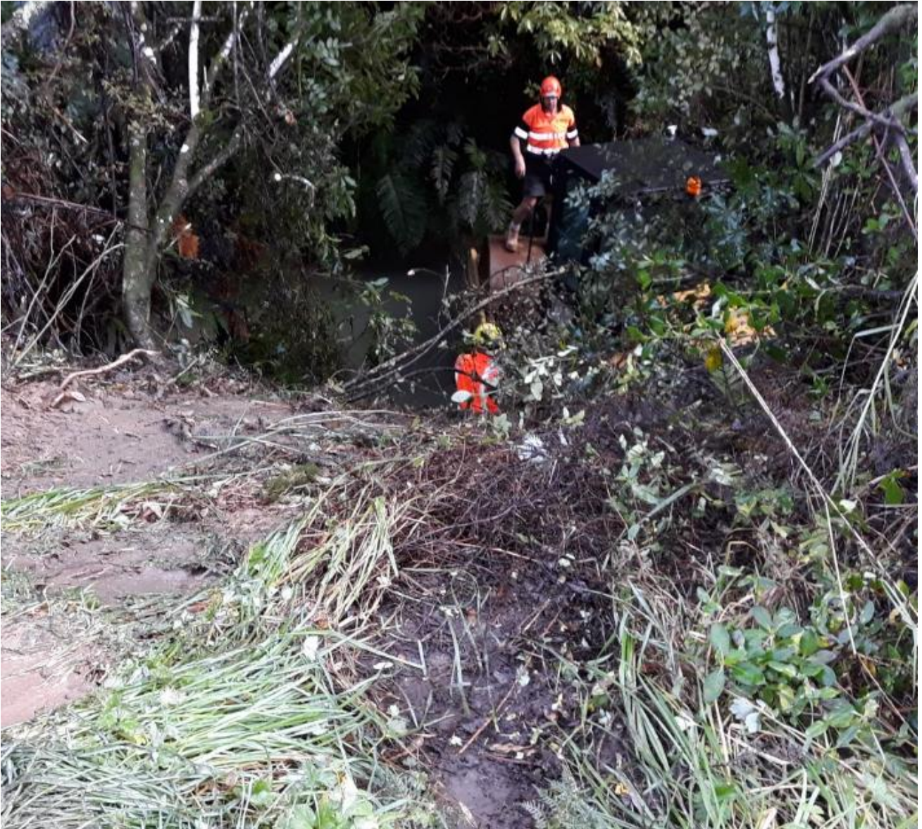
Recovery Team Working on the Roller
