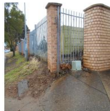
Photo (1a): Work area showing electrical pillar and padmount station
